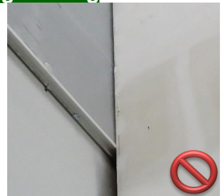
Electrical conduits and insulation panels cannot be within the fire rated joint. The insulation needs to be cut before and after the interior partition.
